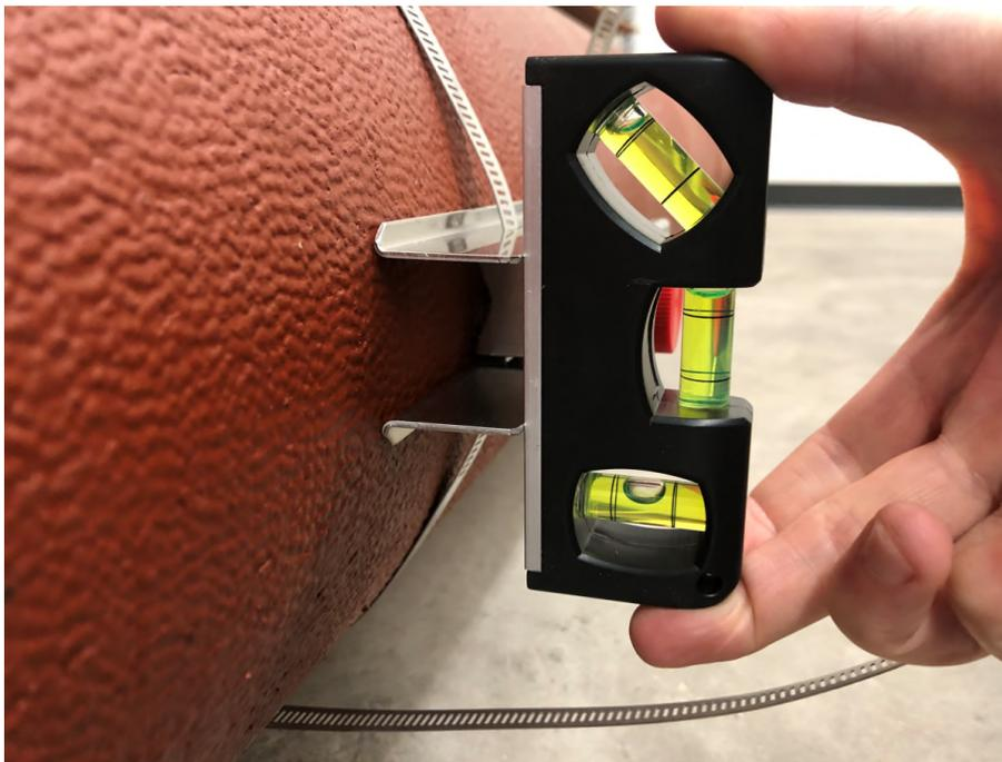
3. Use alignment bar to ensure that the brackets are parallel. Completion of steps 2 and 3 is shown below.
