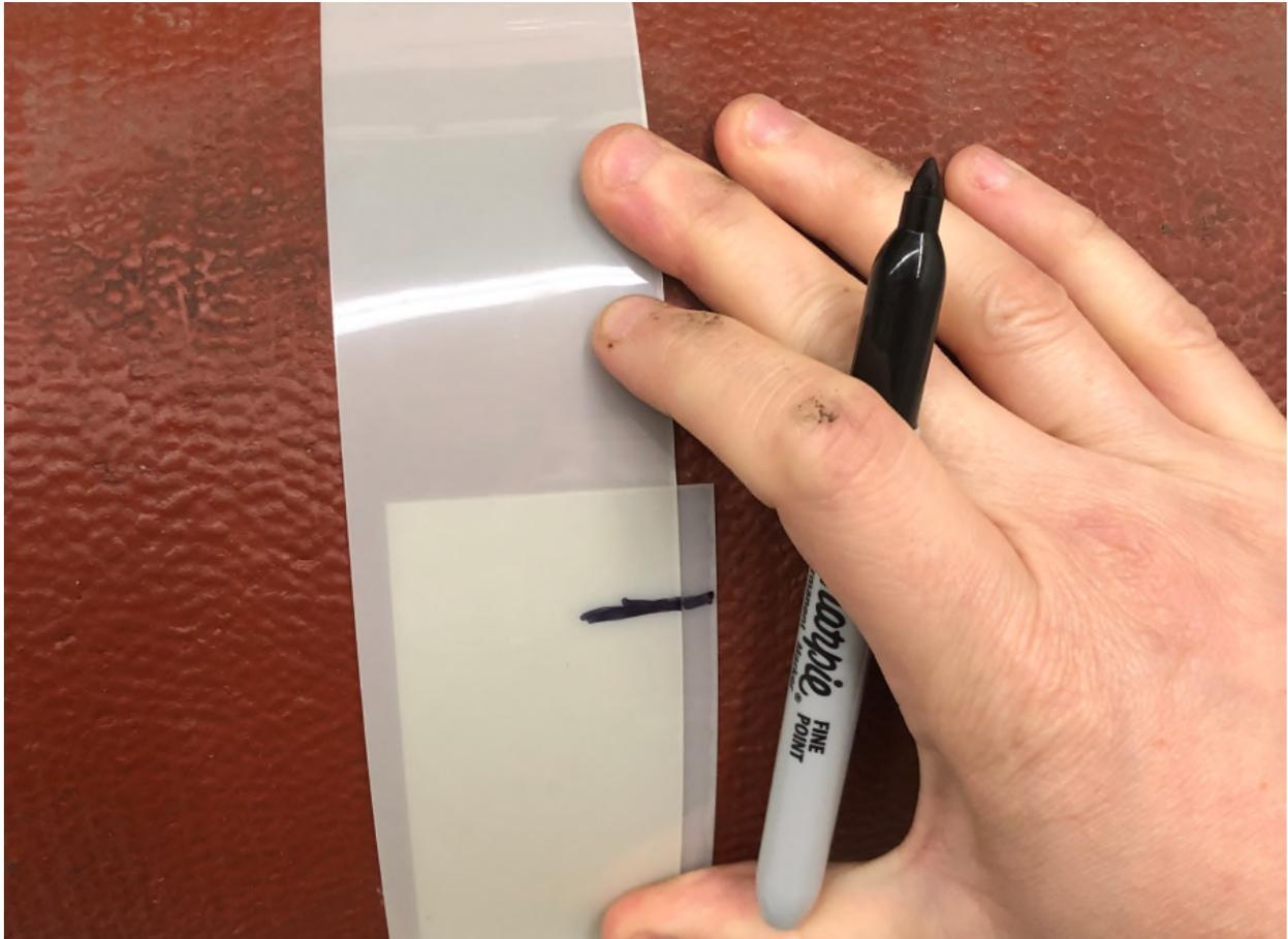
7. Lay the mylar sleeve flat, and use the tape measure to measure half way between the two marks created when you wrapped the mylar around the pipe:
